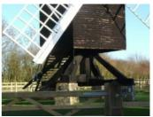
Post mills are so called because a central post supported the whole structure and the whole mill revolved around it.
